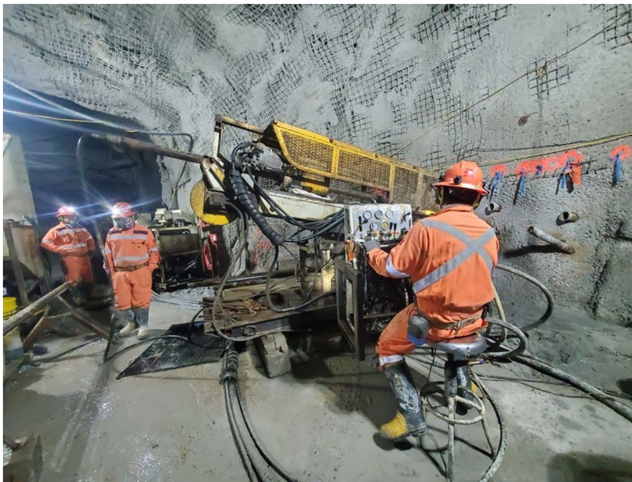
Underground contract drill rig; Level 3 – Arista Mine – Three Sisters / Gloria vein systems
