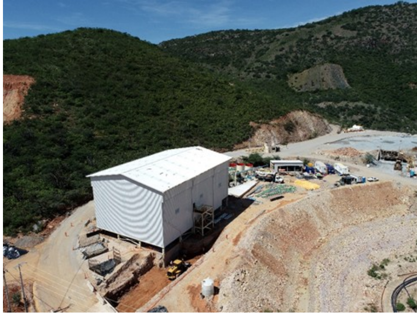
Figure 14-6: DDGM Tailings Filtration Plant.
