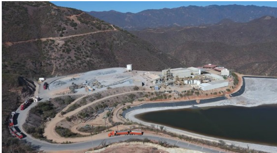
Figure 14-1: The DDGM Processing Facility.
