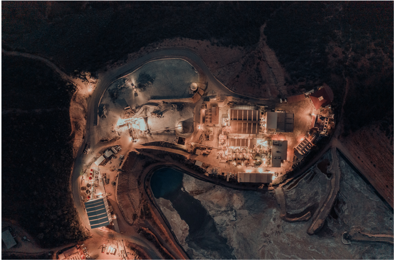
Processing Plant at Night
