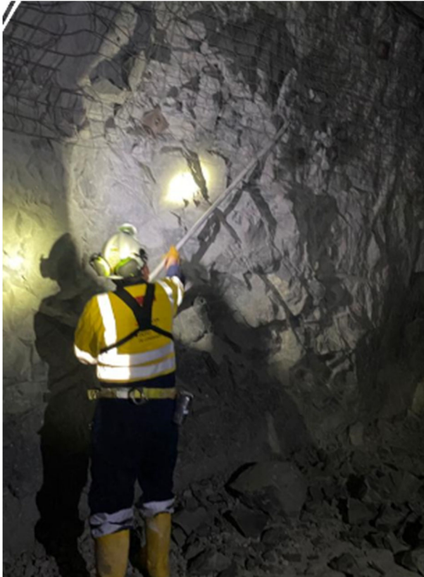
Removing Loose Rock
