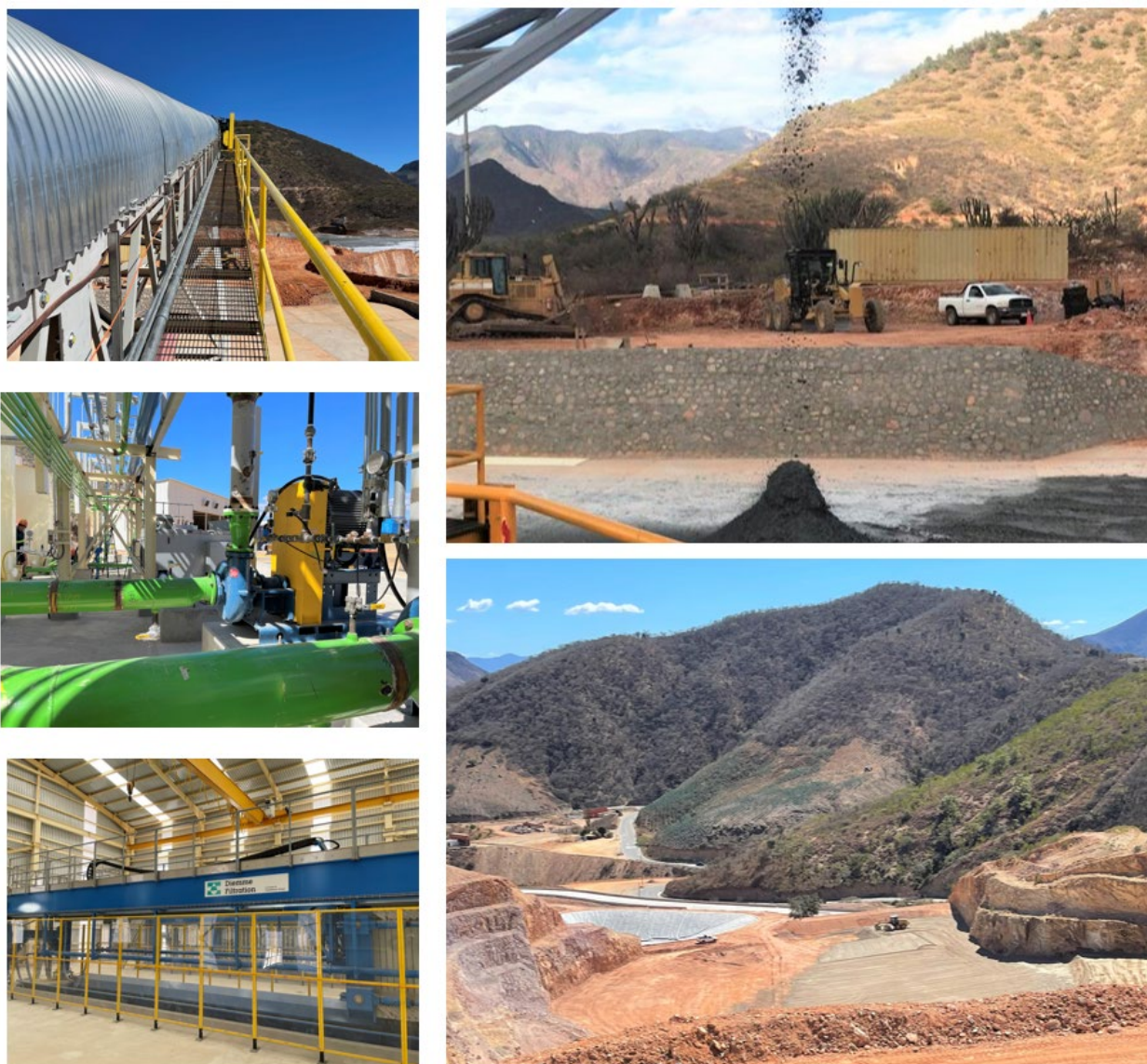
Dry Stack Tailings Filtration Plant and Dry Stack Area
